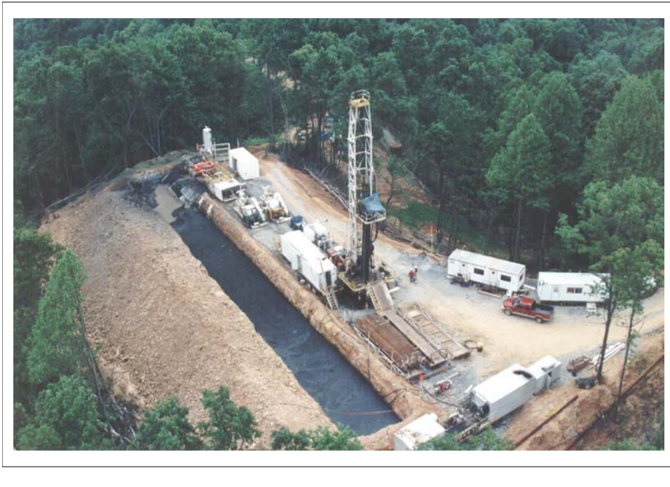
Figure 5: CDX Drilling Rig on Location in the Central Appalachian Basin
